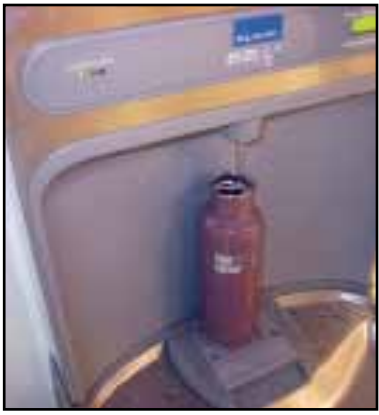
Bottle refilling stations resemble traditional water fountains but offer no-touch refills of filtered water.
